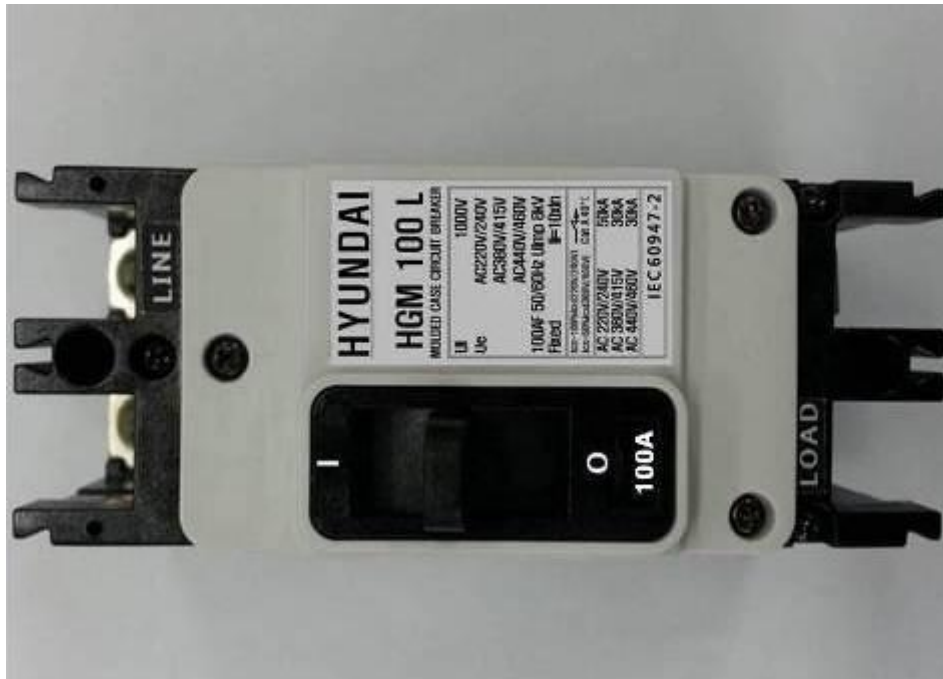
Front view, 2P with fixed thermo-magnetic release, MCCB
